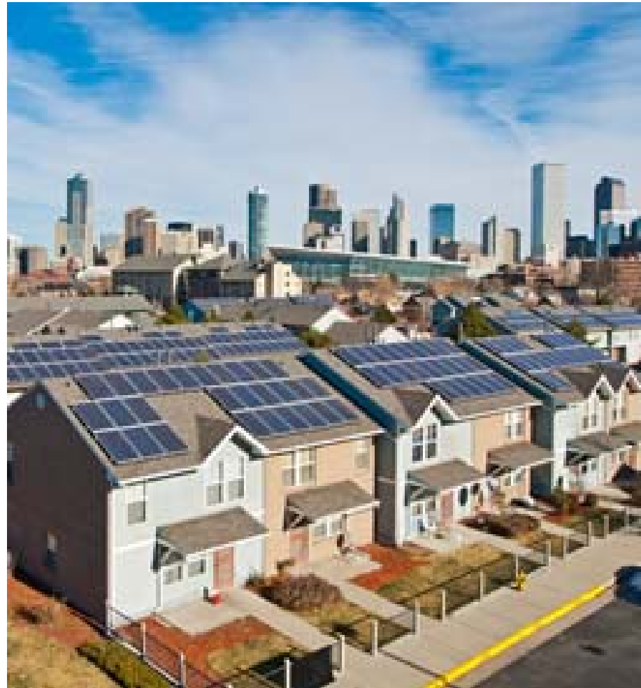
Denver Housing Authority, 2.5 MW Power Purchase Agreement
