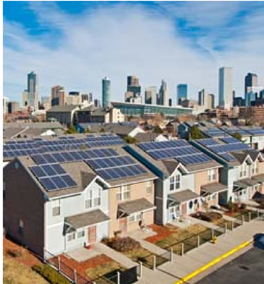
Denver Housing Authority, 2.5 MW Power Purchase Agreement
