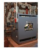
A new 85% AFUE-rated hot water natural gas boiler replaced the existing boiler which had an efficiency of only 60%. The heating efficiency of the house was further improved by increasing the attic insulation from an R-value of 8 to R24, the house was air-sealed and two skylights repaired. Based on before and after blower-door tests, the energy efficient measures installed reduced air-leakage by 30%.
